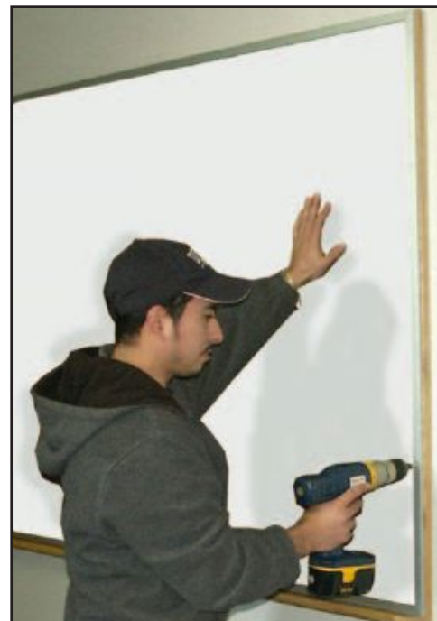
Attach OverBoard with screws through pre-drilled holes in frame
