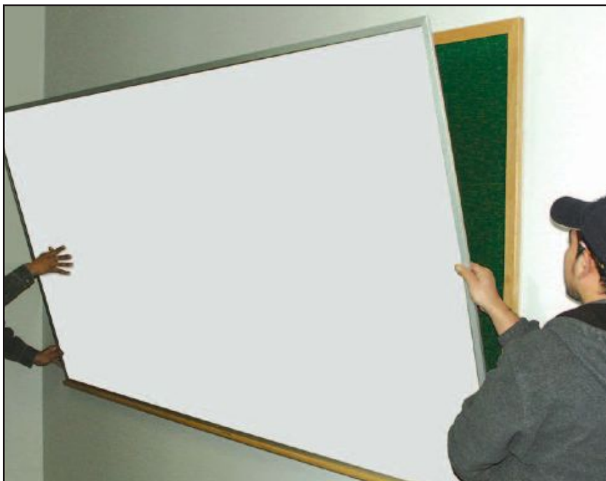
Place OverBoard over existing Board (use adhesive where necessary)
